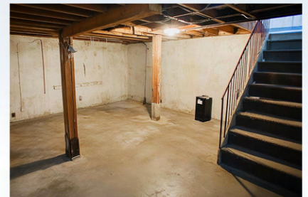
Basements and underground spaces
